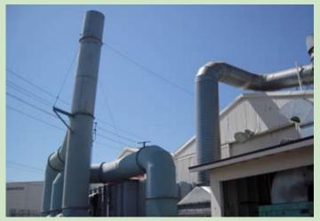
Wilson Partitions' paintline system captures 100percent of VOCs from the paint as aluminum extrusions are process. The VOC's are funneled into a thermal oxidizers which then destroy 99.3percent of all VOCs.
